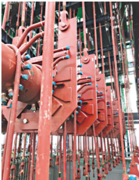
Combine Masinloc power plant project
